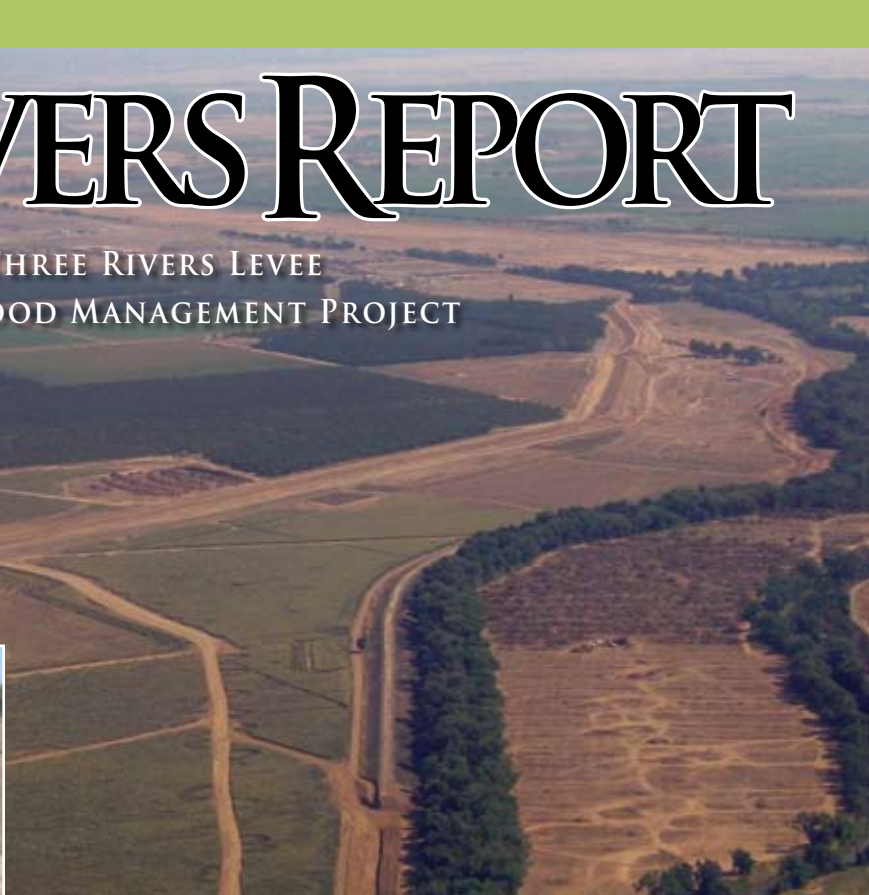
Aerial view of the Bear River Setback Levee
