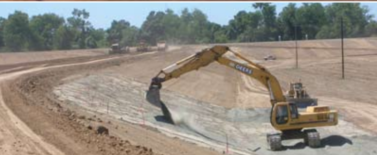
Construction of Bear River Levee
