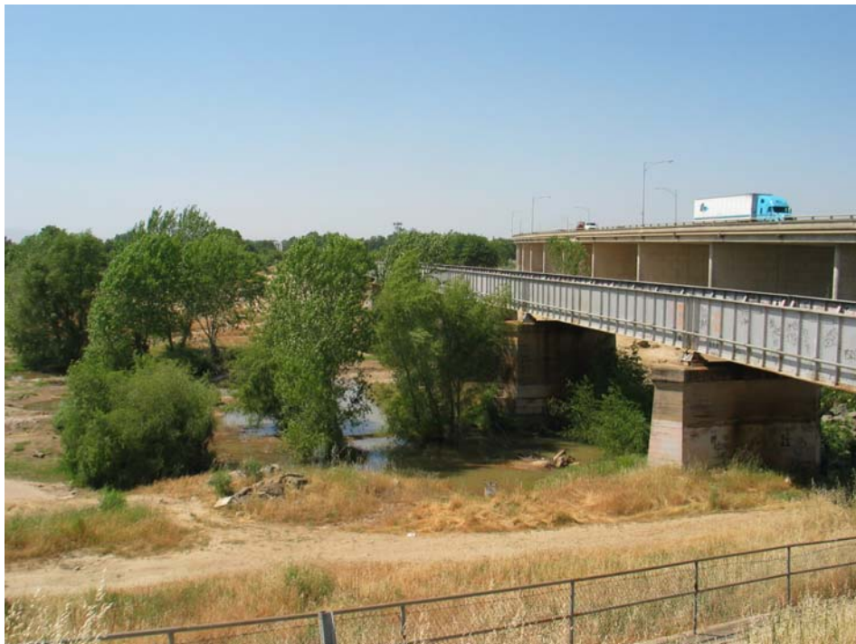
B. SR 70 and railroad bridge adjacent to the project area. View to the north from the existing Feather River levee at the northern end of Segment 3.
