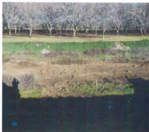
Backfill of Plant Excavation
