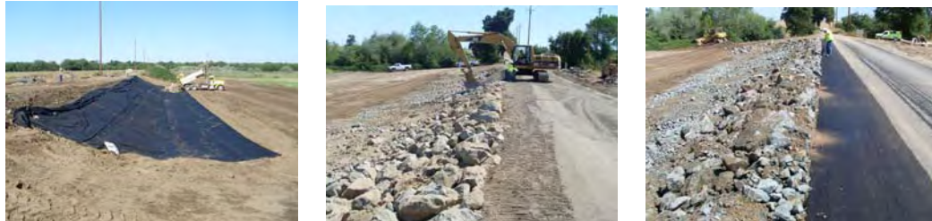
Repair of abandoned Country Club Road in Setback Area
