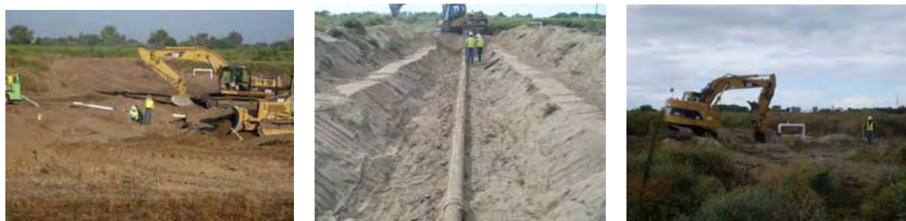
Asbestos Pipe Removal from Feather Setback Area
