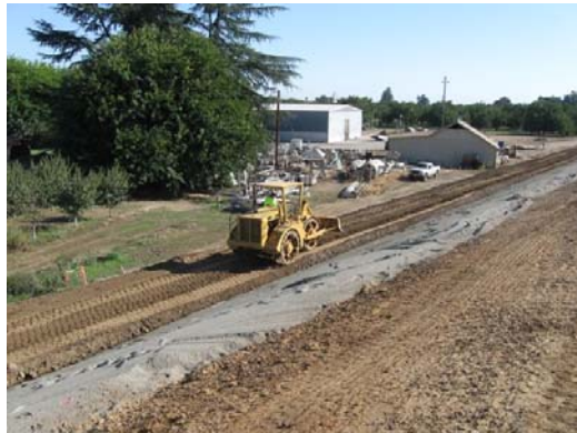
Crack Repair – Feather Segment 1
