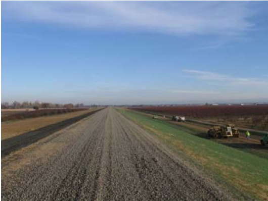
Completed Feather Setback Levee
