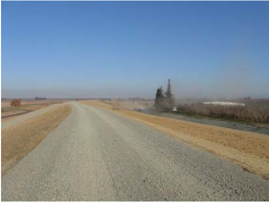
Completed Feather Setback Levee
