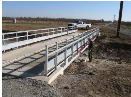
Bridge over landside drainage channel
