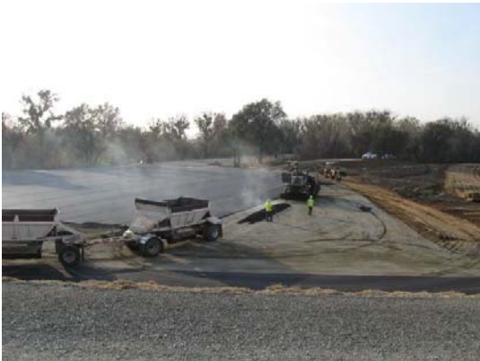
Star Bend Parking lot
