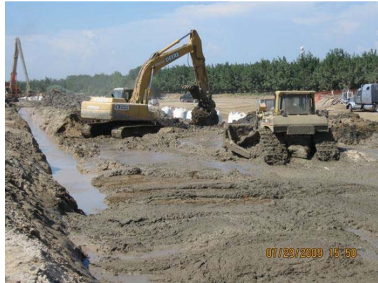
Slurry Wall @ South Tie-In
