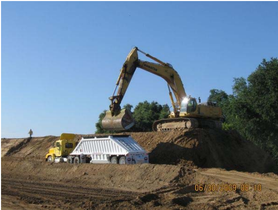
Existing Levee Work @ South Tie-In Sept - South Tie-In Levee @ Cultural Site
