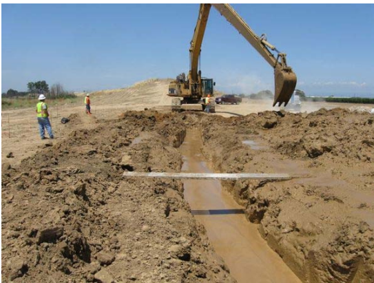
Slurry Wall Construction
