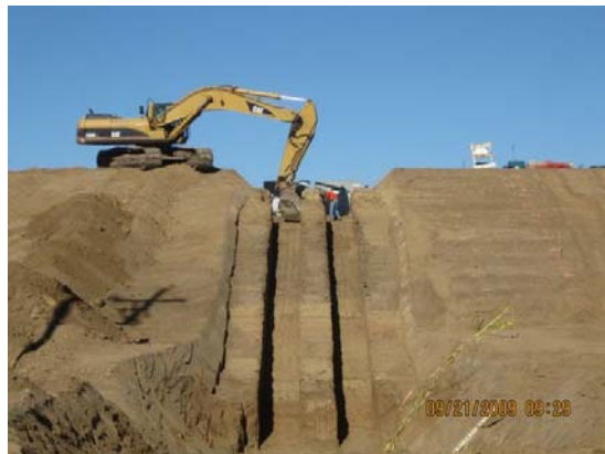
Pump Station 3 pipe Alignment Over levee
