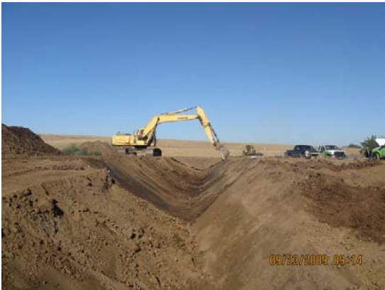
Landside Drainage Ditch
