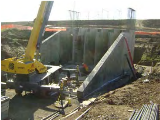
January New Pump Station # 3
